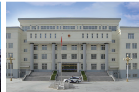
Gansu Jingning conservancy bureau
