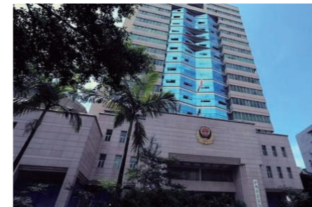
Luzhou police office building
