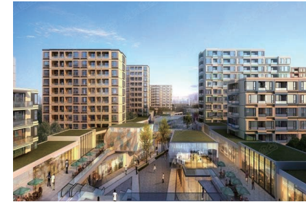
Greentown Foshan Yangliu County
