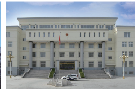
Gansu Jingning conservancy bureau
