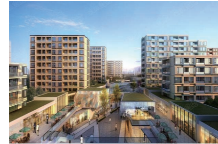
Greentown Foshan Yangliu County
