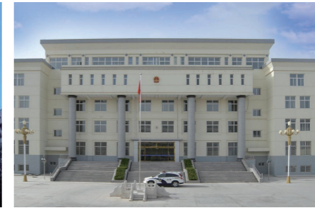
Gansu Jingning conservancy bureau
