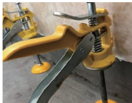
Multiple height lifters need to be placed, one for a distance of about 30 centimeters
