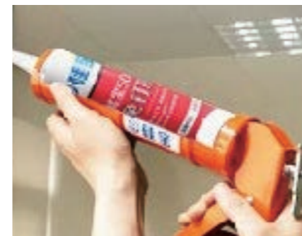
Cut the rubber bottle and install the rubber nozzle Install the glue gun and press the handle of the glue gun
