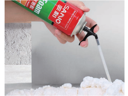
Two-thirds of the spray filling area is sufficient
