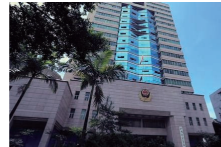
Luzhou police office building
