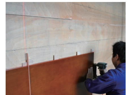
Aim the gun head at the position where the nail is to be nailed and then pull the trigger
